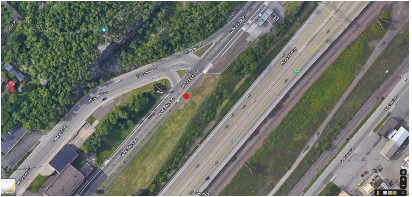
Lincoln Park Solar Project site
